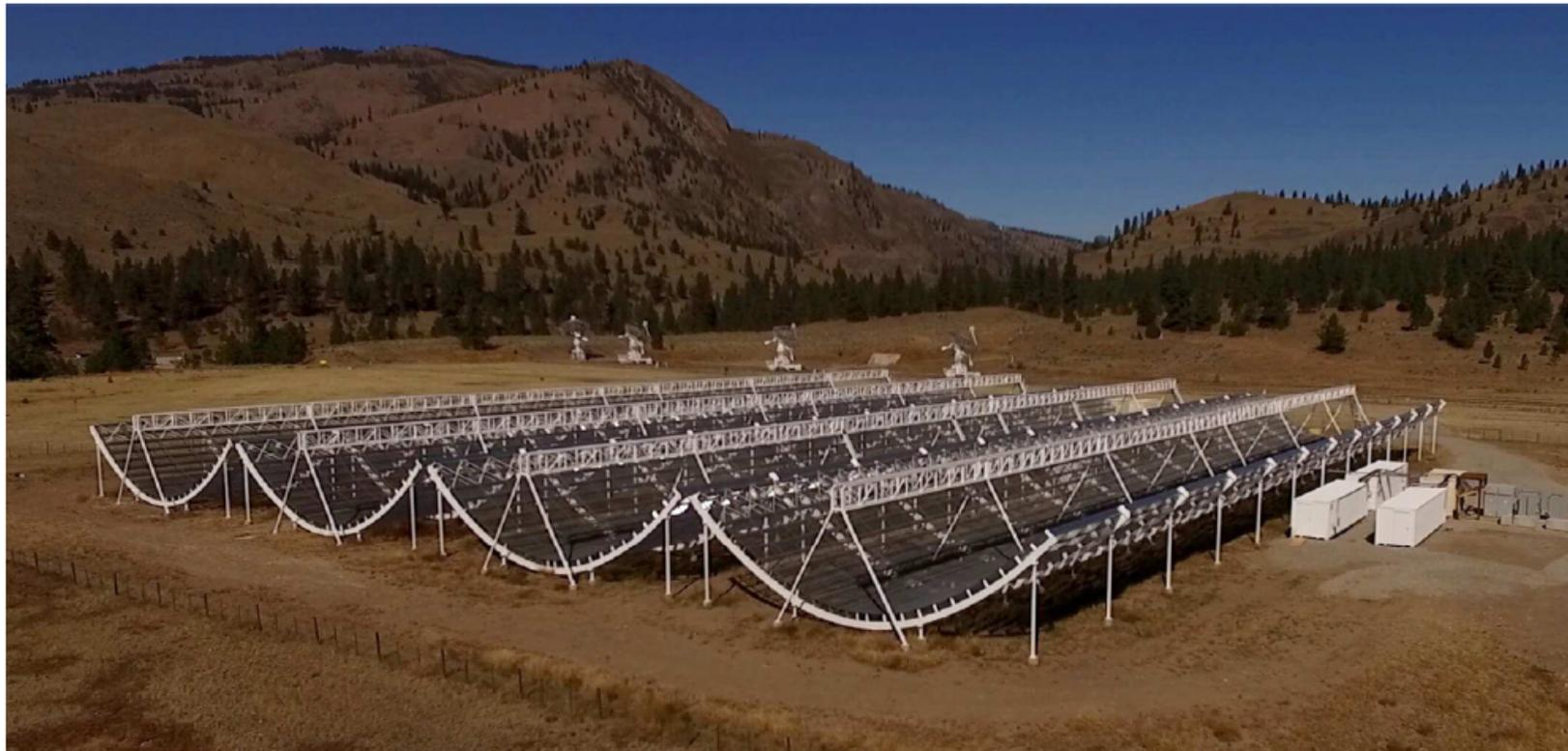
**Figure 1.** Photograph of the CHIME telescope on 2016 September 15, looking northwest. The shipping containers housing the X-Engine and CHIME/FRB back end can be seen adjacent to the rightmost cylinder. The receiver huts containing the F-Engine are beneath the reflectors and cannot be seen here. The DRAO Synthesis Telescope (Kotthes et al. 2010) can be seen in the background. See Table 1 for detailed properties of CHIME.
